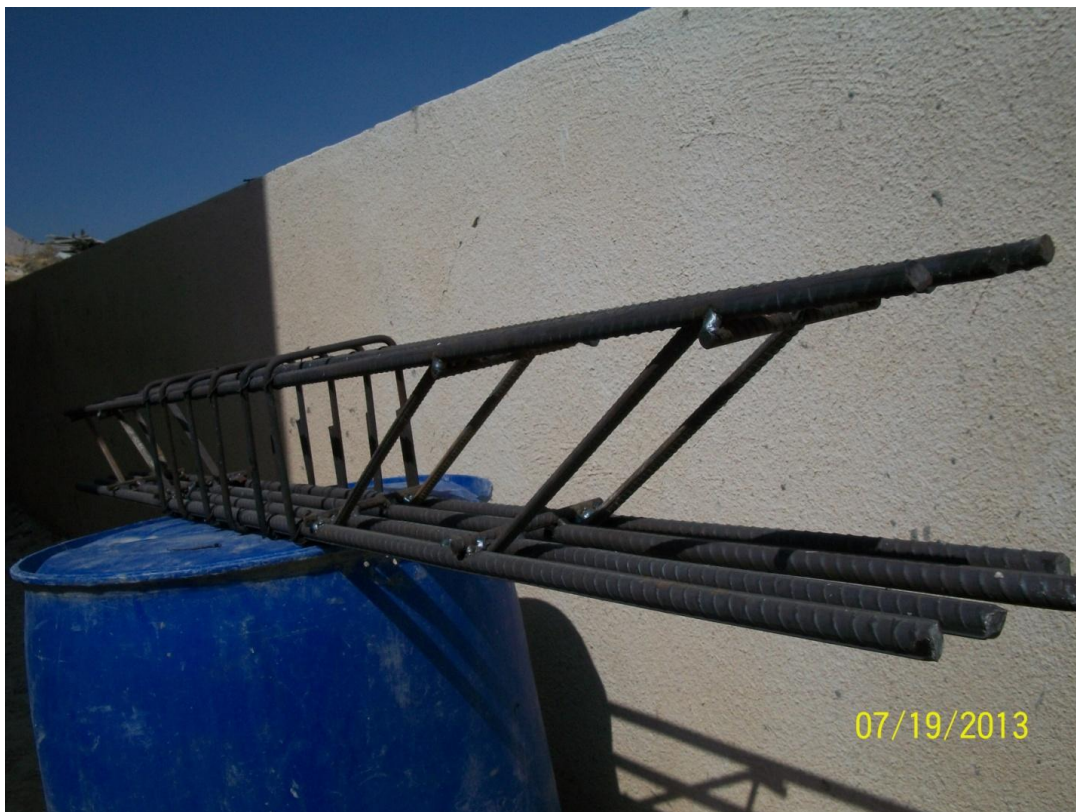
Figure 2: Steel cage reinforcement of the beam BW, welded swimmer bars.
