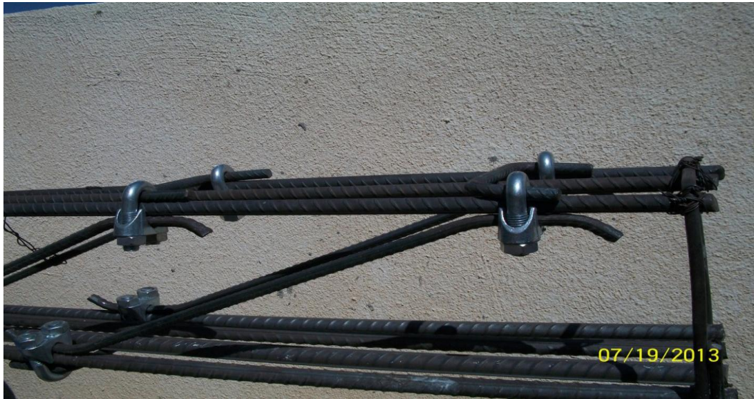
Figure 3: Steel cage reinforcement of the beam, BU, U-link bolted swimmer bars.
